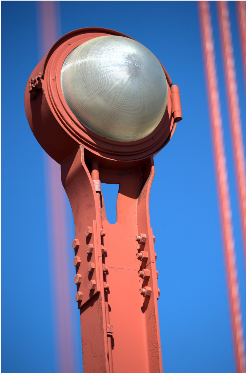
Abb. 143 Detail der Golden Gate Bridge
