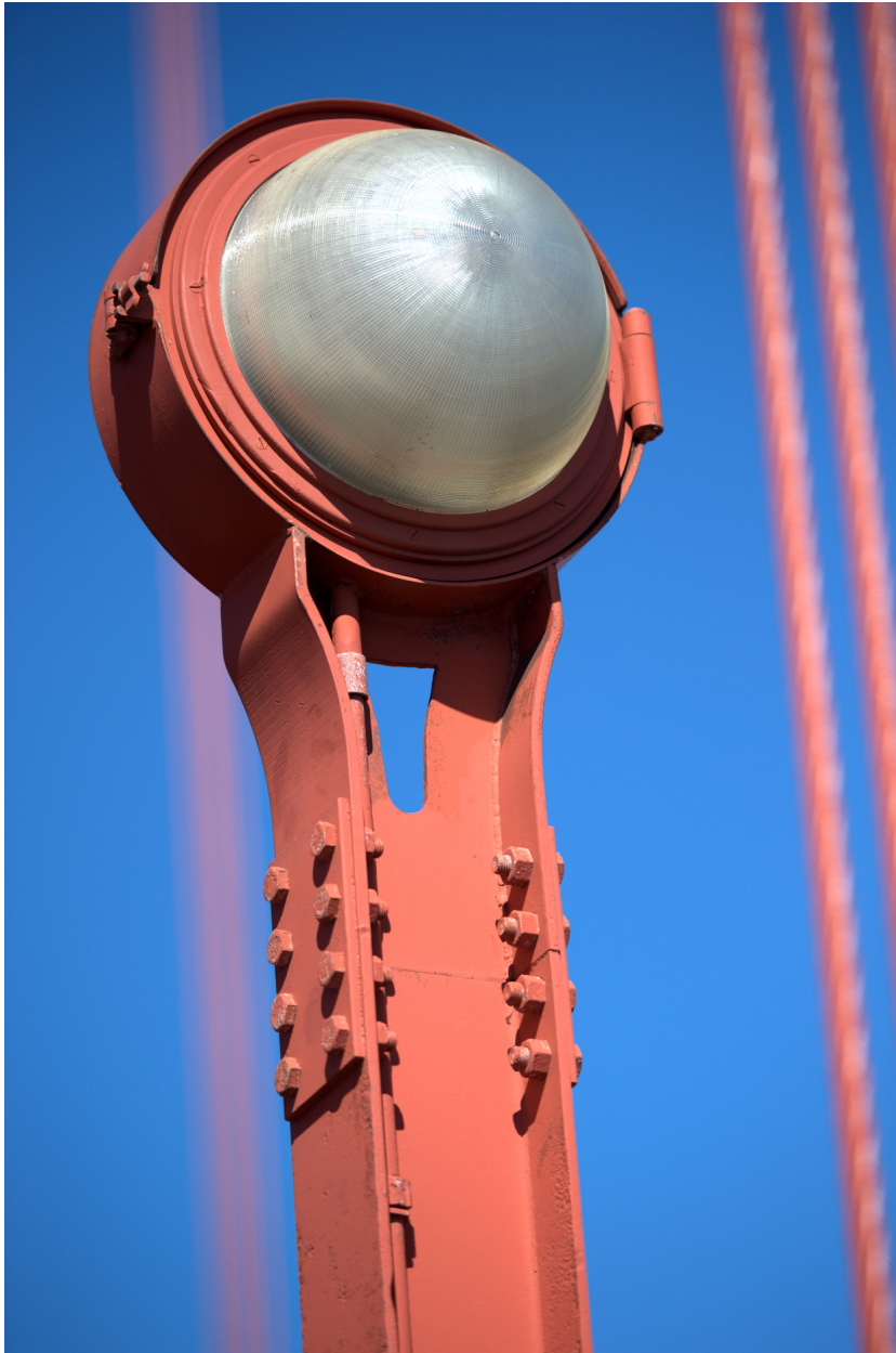
Abb. 133 Detail der Golden Gate Bridge
