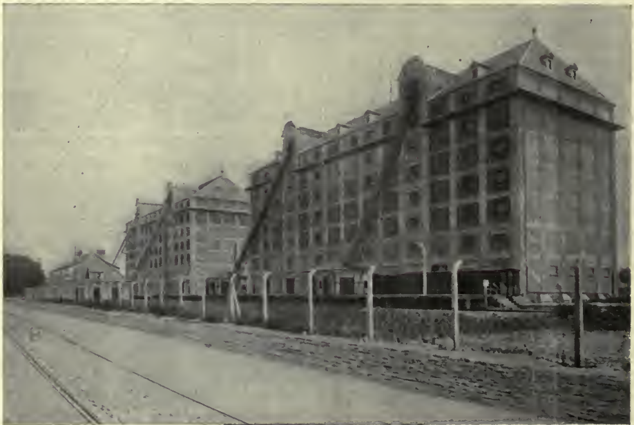
The RUSSEHHOFS. — Note the four electrically driven elevators. Discharging from cars.
