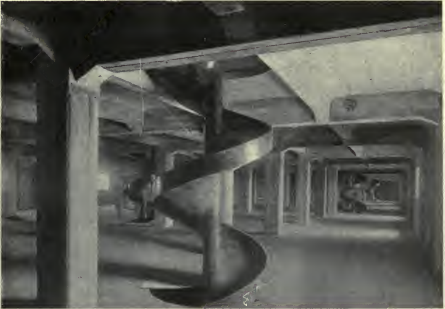
The spiral chutes for sack goods in the RUSSENHOFS.
