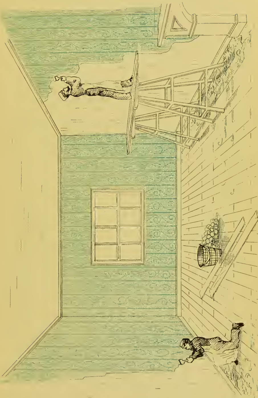
Stripping poisonous wall papers.
