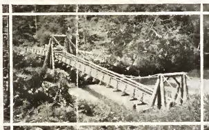
Thunder Creek suspension bridge
