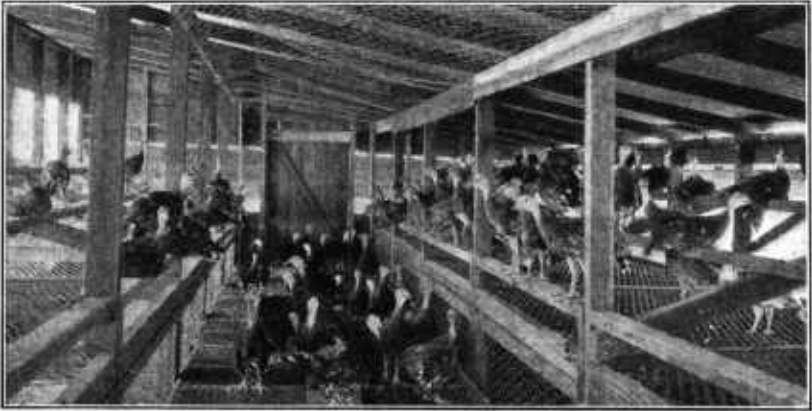
FIGURE 20.—Interior of 16 by 25 foot range house showing wire floor and wire under roosts
