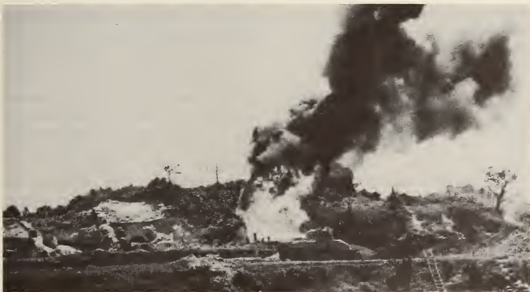
BLOWTORCH: A flame tank burns out Japanese positions in hillside tombs during the drive for Naha. (USMC 122153)
