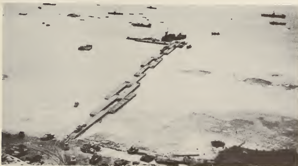
CAUSEWAYS relieve logistical problems as tons of supplies are transported inland. (USMC 118304)
