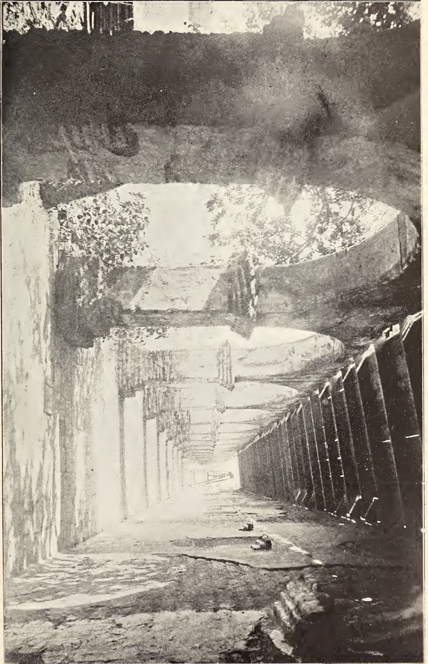
INNER CLOISTERS, SAN JUAN CAPISTRANO. (Re-roofed by the Landmarks Club.)
