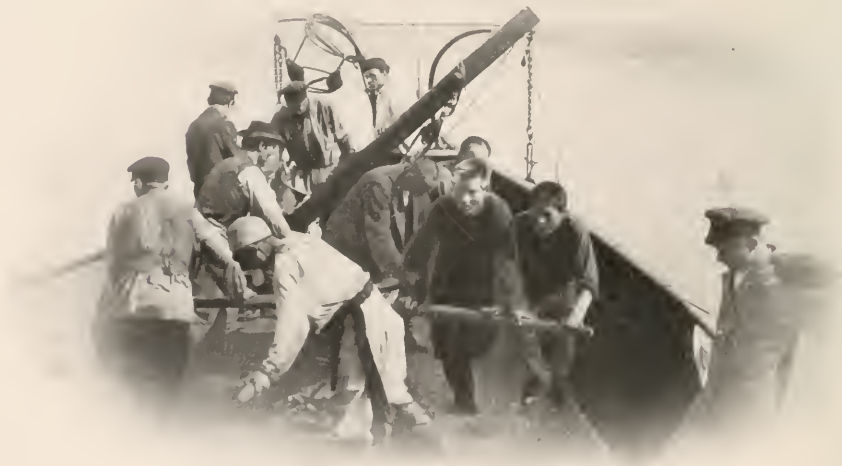
WORKING THE WINCH
