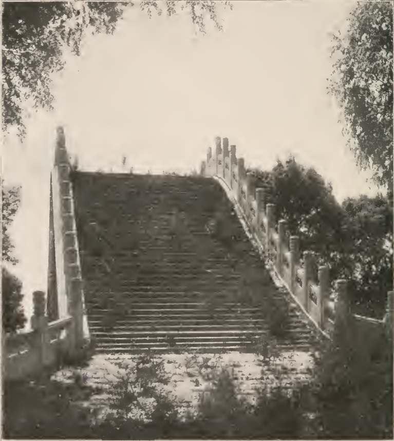
THE STAIRWAY OF THE MARBLE BRIDGE
