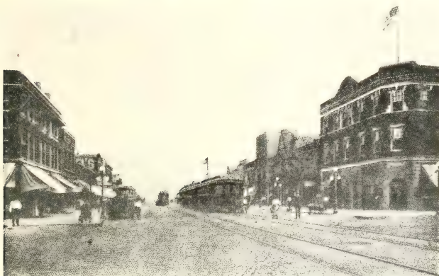
CHICAGO AVENUE EAST OF FORSYTH AVENUE
