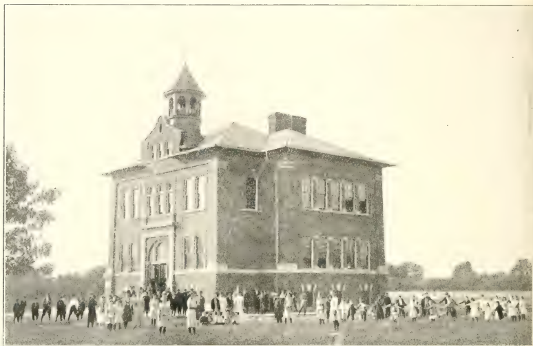
SHELBY CONSOLIDATED SCHOOL, CEDAR CREEK TOWNSHIP
