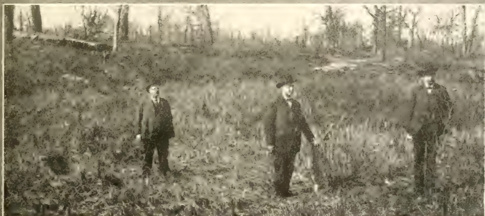
ABOUT TO BREAK GROUND AT GARY
