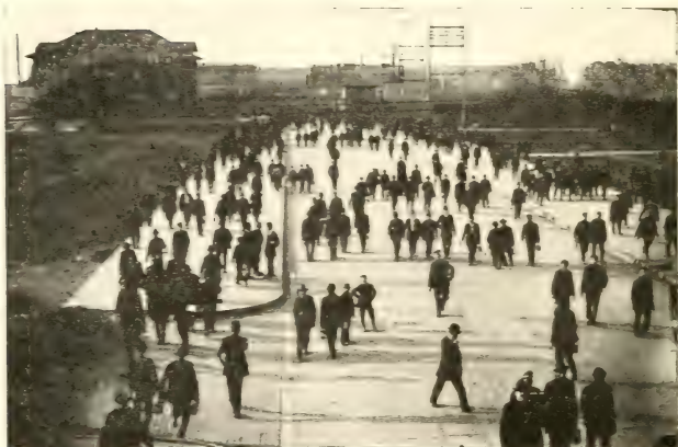
UP BROADWAY TOWARD THE STEEL MILLS
