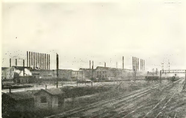
VIEW OF INDUSTRIAL SECTION
