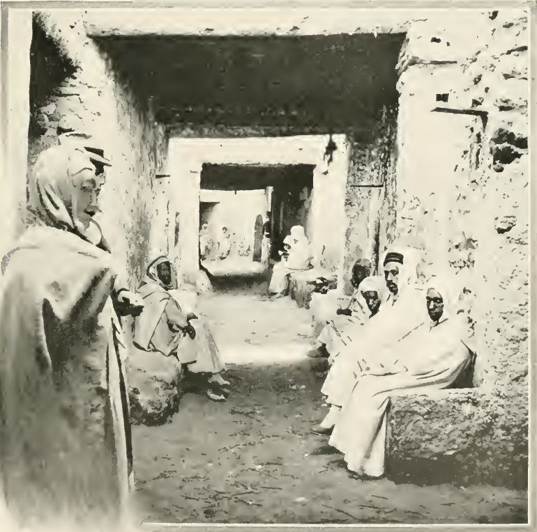
THE TUNNEL-LIKE STREETS OF TOUGGOURT
