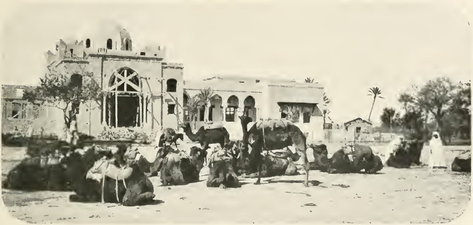
THE CASINO IN CONSTRUCTION
