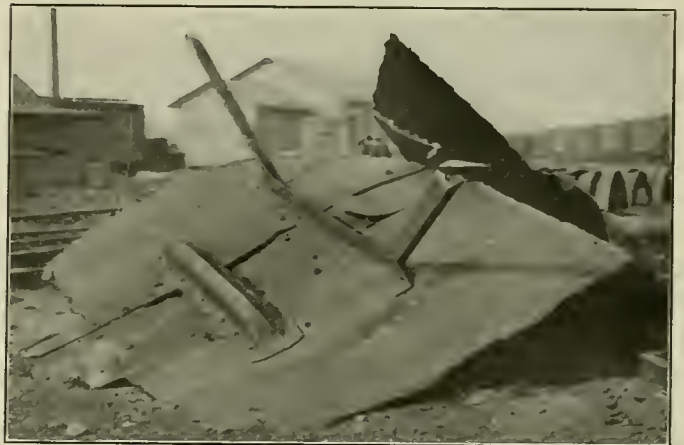
Fig. 8—Rusted Floor Sheet Cut from a Hopper Coal Car with a Broad Axe as Shown in Fig. 9
