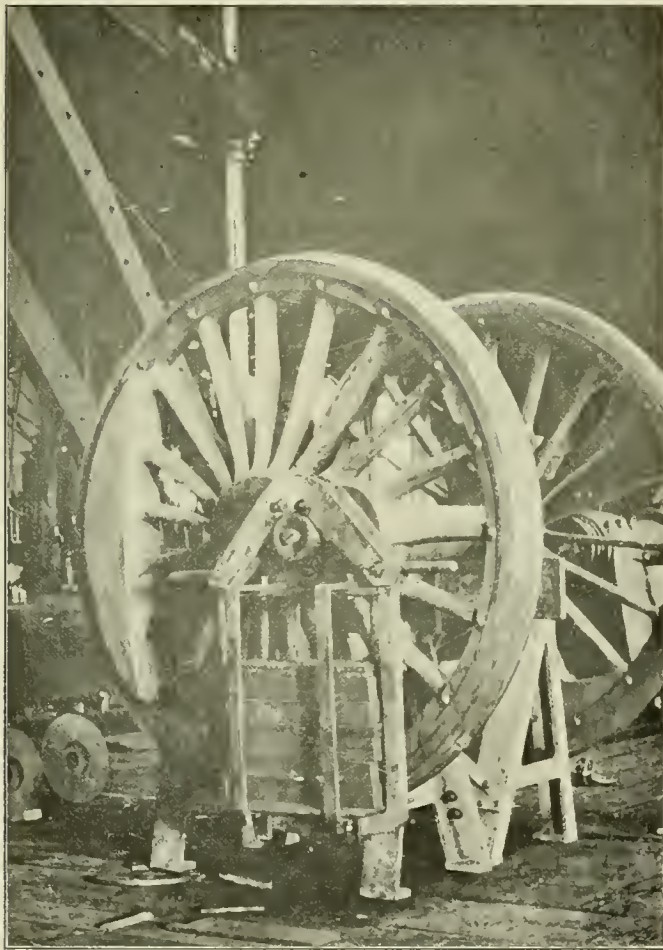
Fig. 1—Adjusting Counterbalance on a Locomotive
