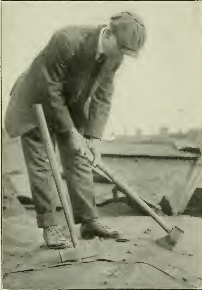
Fig. 9—Broad Axe Made by Drawing Out One End of a Sledge, and the Manner of Using It to Cut Rusted Steel Sheets
