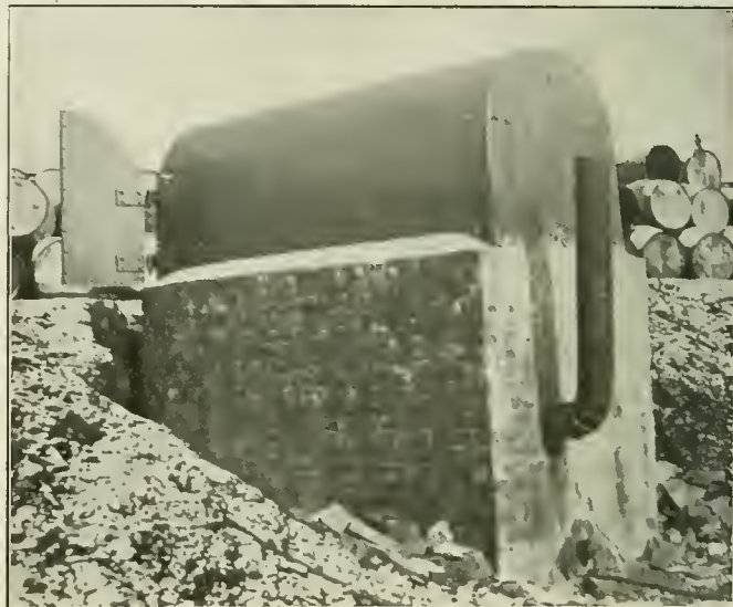
Furnace for Melting Heavy Oil from Sides of Metal Barrels
