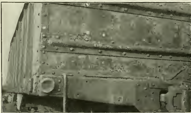
Fig. 3—A Steel Car Five Years Old in Which the Hopper Sheets Required Renewal on Account of Corrosion; Note the Rusted Condition of the End, Stiffening Rib and Buffer Plate
