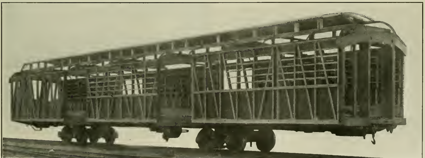
The Body Framing of the Baggage Cars
