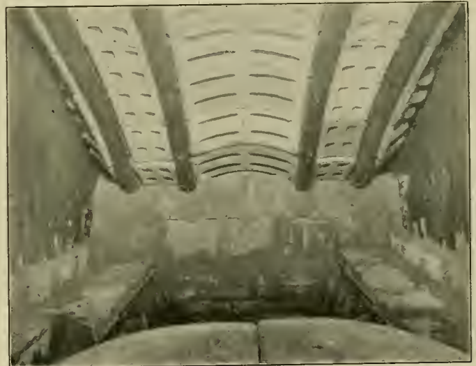
Looking Forward in the Firebox of the Pulverized Fuel Locomotive
