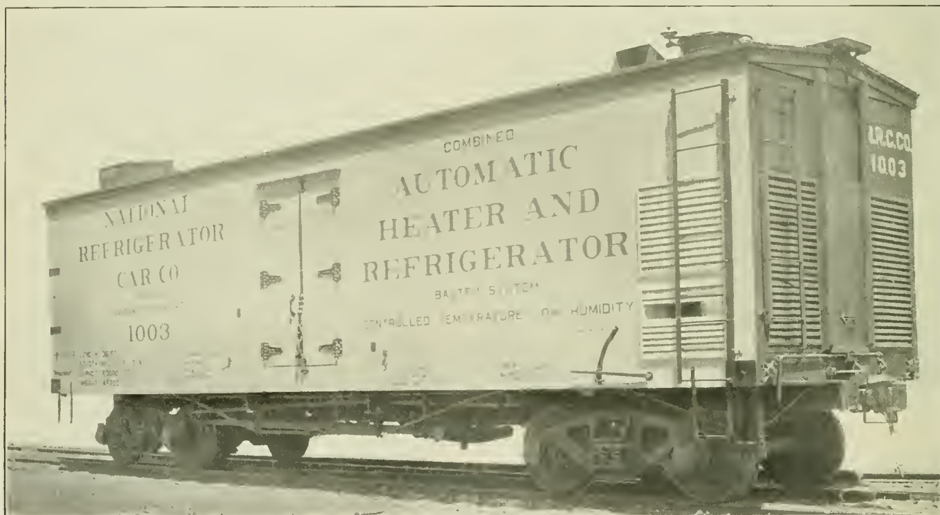
Automatic Refrigerator and Heater Car Which Uses the Ammonia Absorption Process
