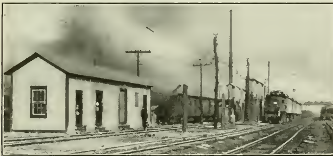
Locomotive Inspection Facilities at Bluefield; a Pit, Which Cannot be Seen is Located in the Second Track in Front of the Frame Building
