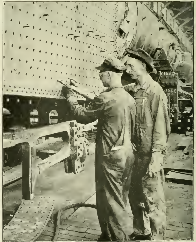
Instructing a Boilermaker Apprentice on Staybolt Work
