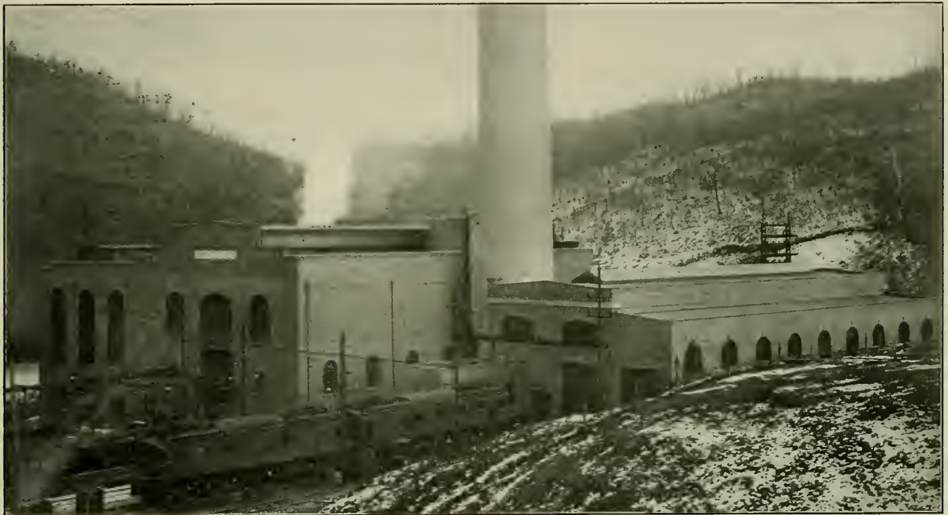
Power House and Locomotive Inspection Building at Bluestone
