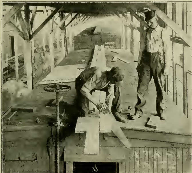
Freight Car Apprentice Repairing a Car Roof
