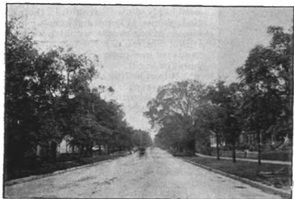
SECOND STREET PAVED WITH SHELL CONCRETE.
