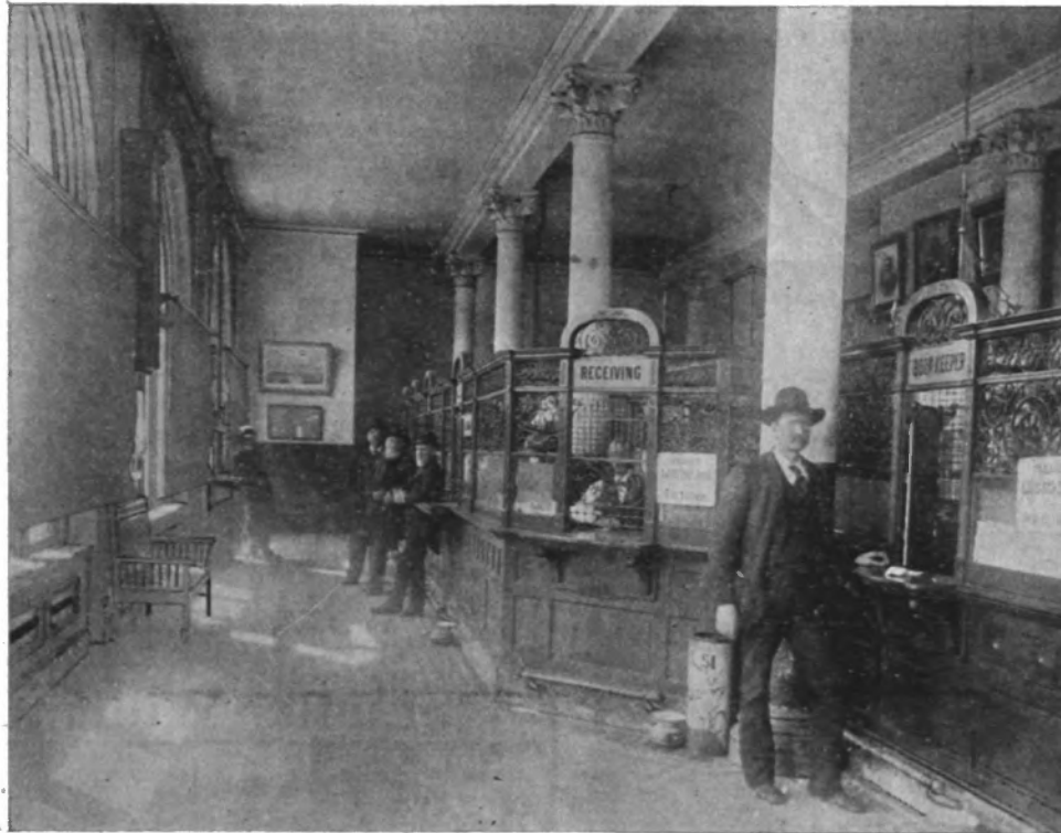
INTERIOR OF EXCHANGE BANK.
