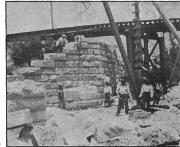
BUILDING TRESTLE ON M. & N. R. R., NEAR MADISON.
