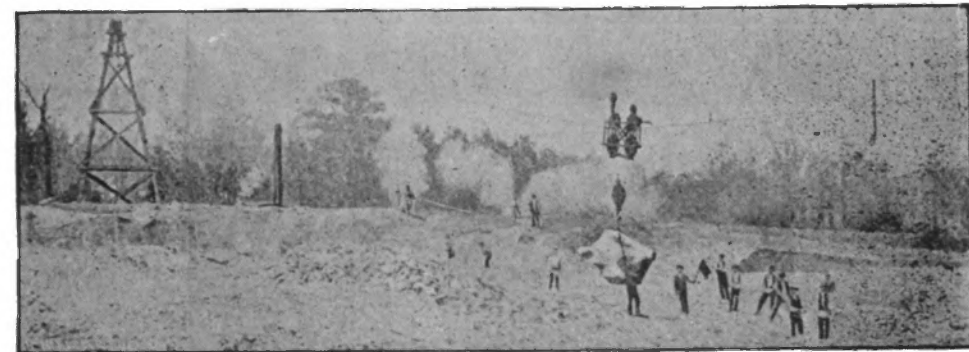
GEORGIA-QUINCY GRANITE CO'S. QUARRY NO. 4.—Loading large jetty stone with Locke-Miller cableway. Cable carrying a 6-ton stone.
