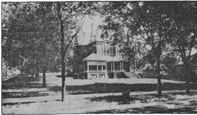
RESIDENCE OF S. R. JAQUES.
