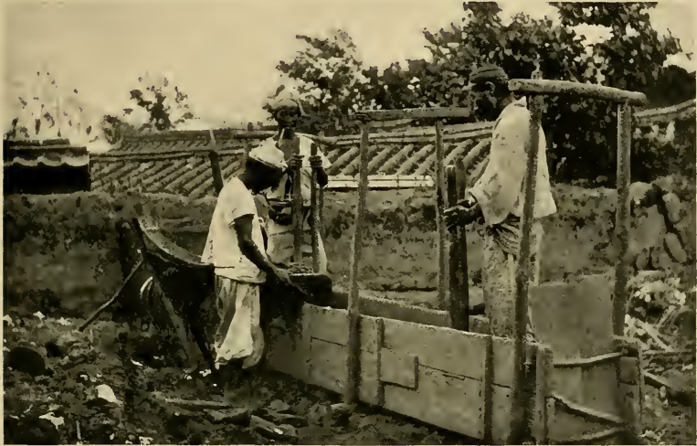
BRICK LAYING EXTRAORDINARY
