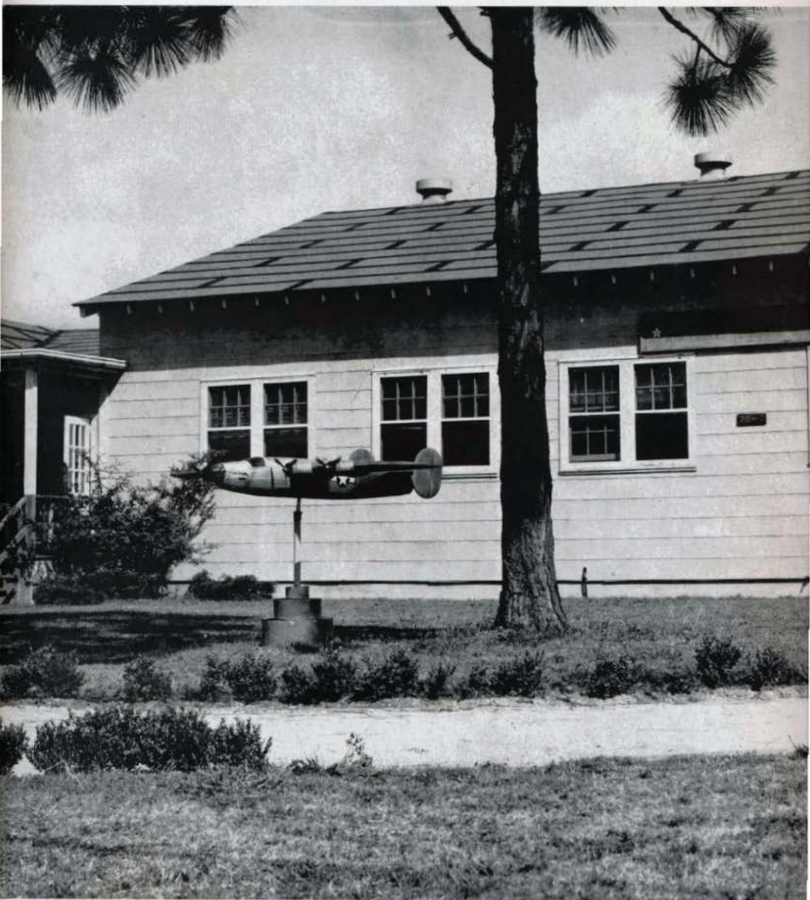
TECHNICAL SCHOOL HEADQUARTERS BUILDING
