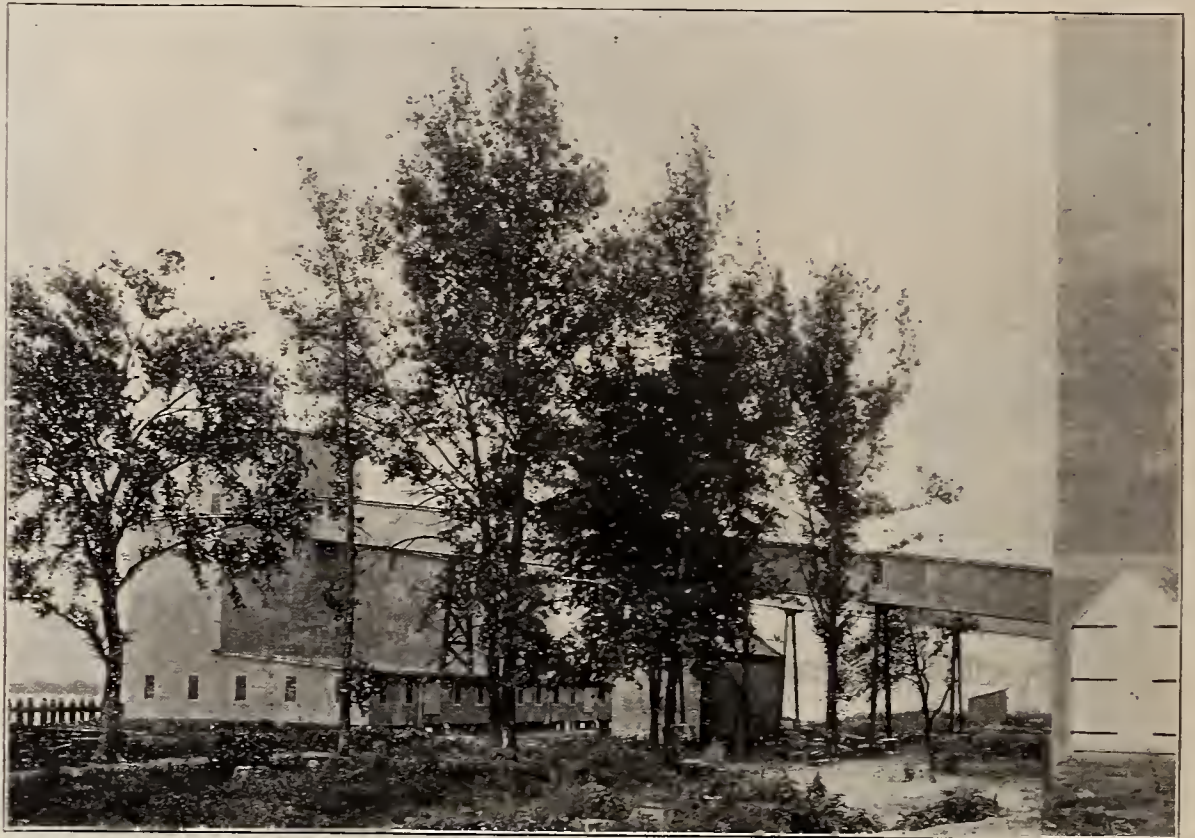
RIVER HOUSE AND BELT GALLERY OF THE BURLINGTON ELEVATOR.
