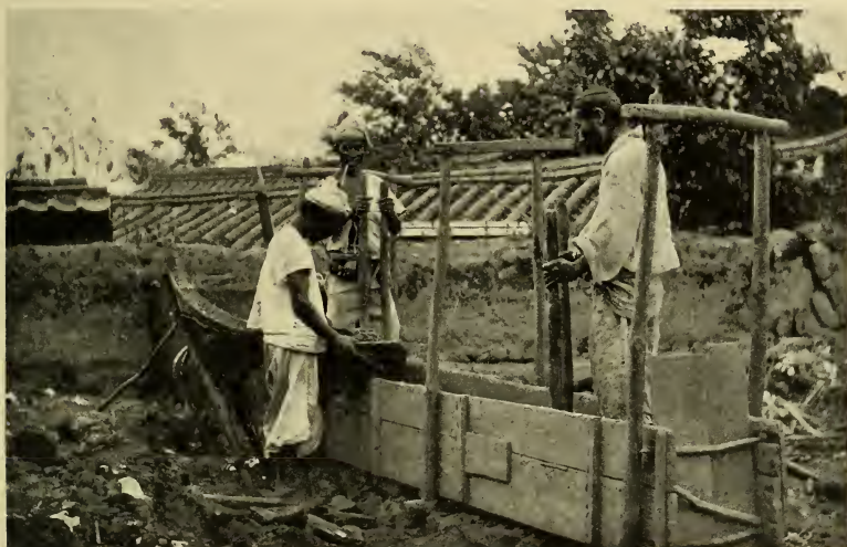
BRICK LAYING EXTRAORDINARY
