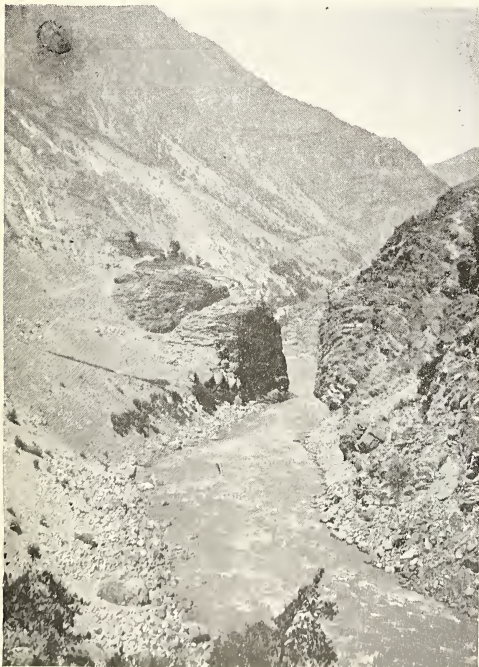
Fig. 7.—The Bridge over the Sutlej between Poo and Namgia.
