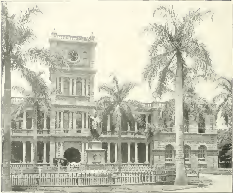
THE GOVERNMENT BUILDING
