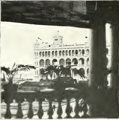
A NEW BUILDING
