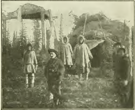
Native Igloo, with Scaffold for Stores.
