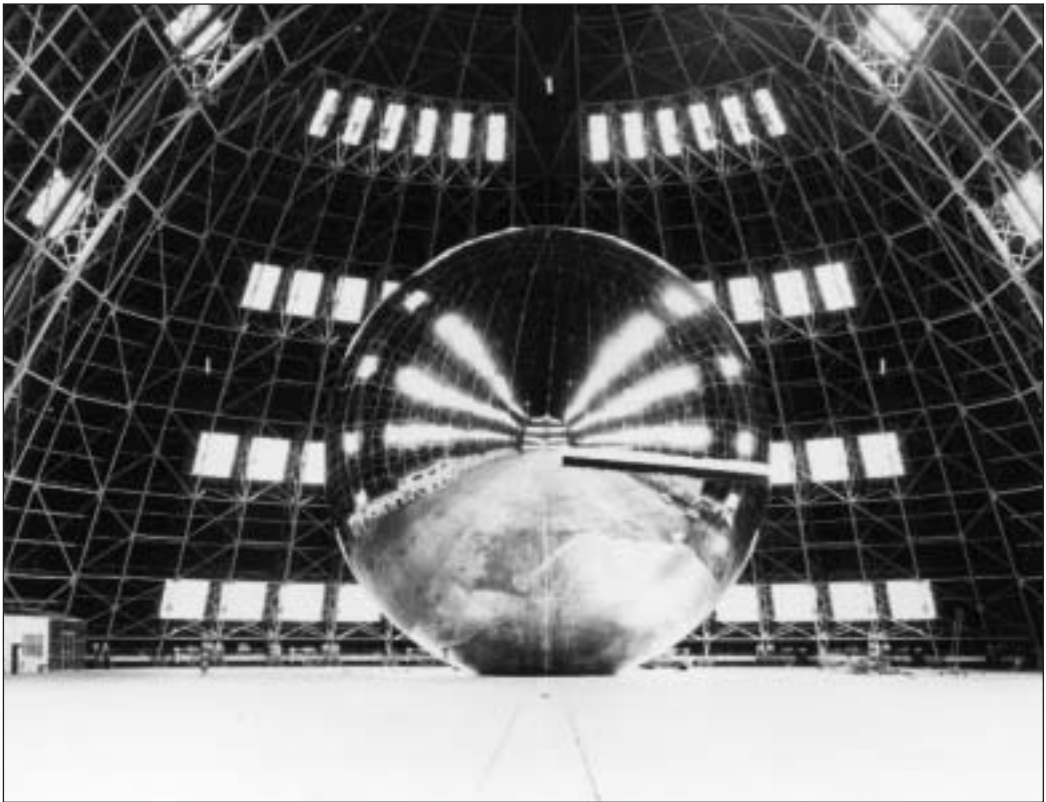
Plastic sphere, 100 feet in diameter, of [the] type to be used in satellite transmission experiments. In orbit, thin plastic with aluminized surface will reflect microwaves.
