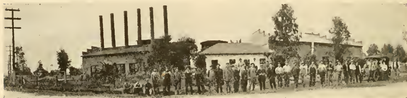
PIPE LINE PUMPING STATION, CORCORAN, CAL.
