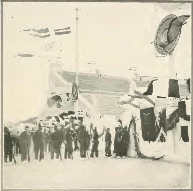
ENTRANCE FOR THE PUBLIC
