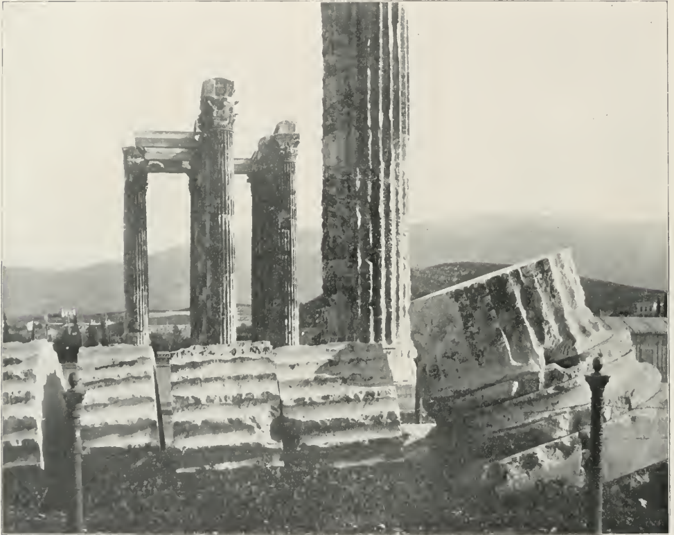
A FALLEN COLUMN
