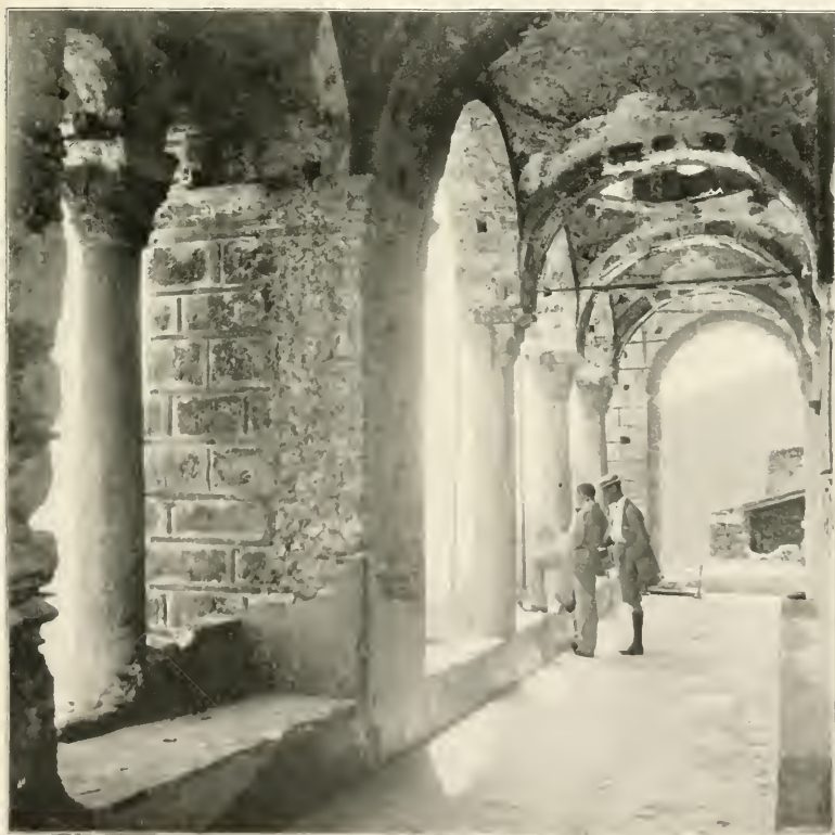
SUNSHINE AND DESOLATION
