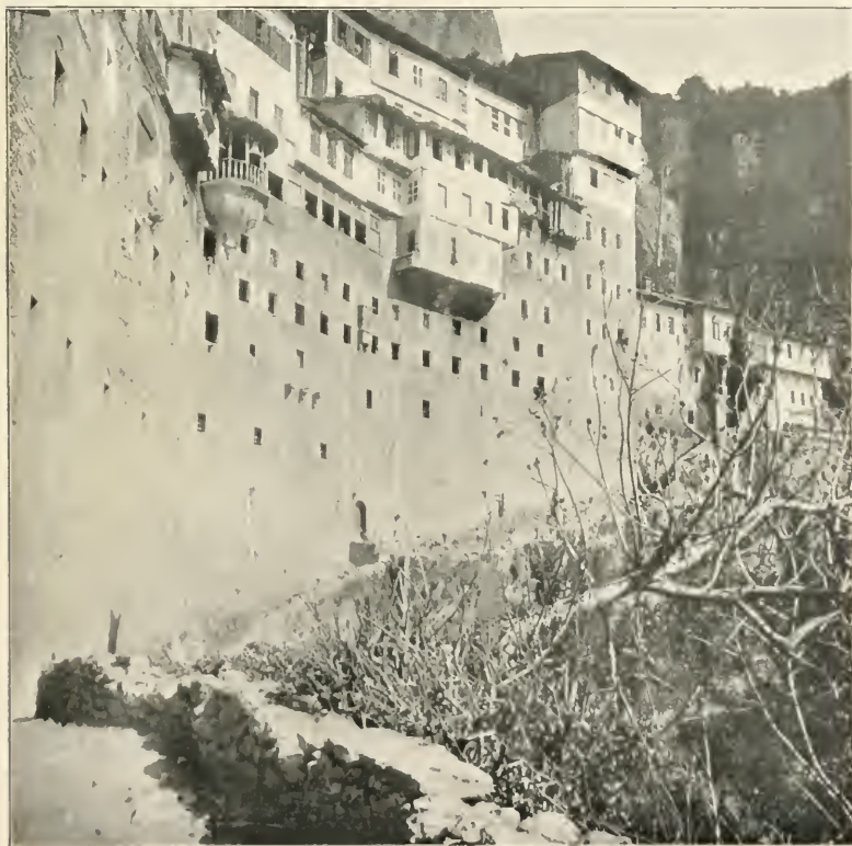
THE CELLAR WALLS
