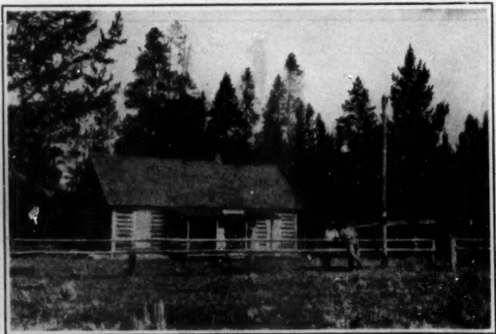
A Ranger Station in Wyoming
