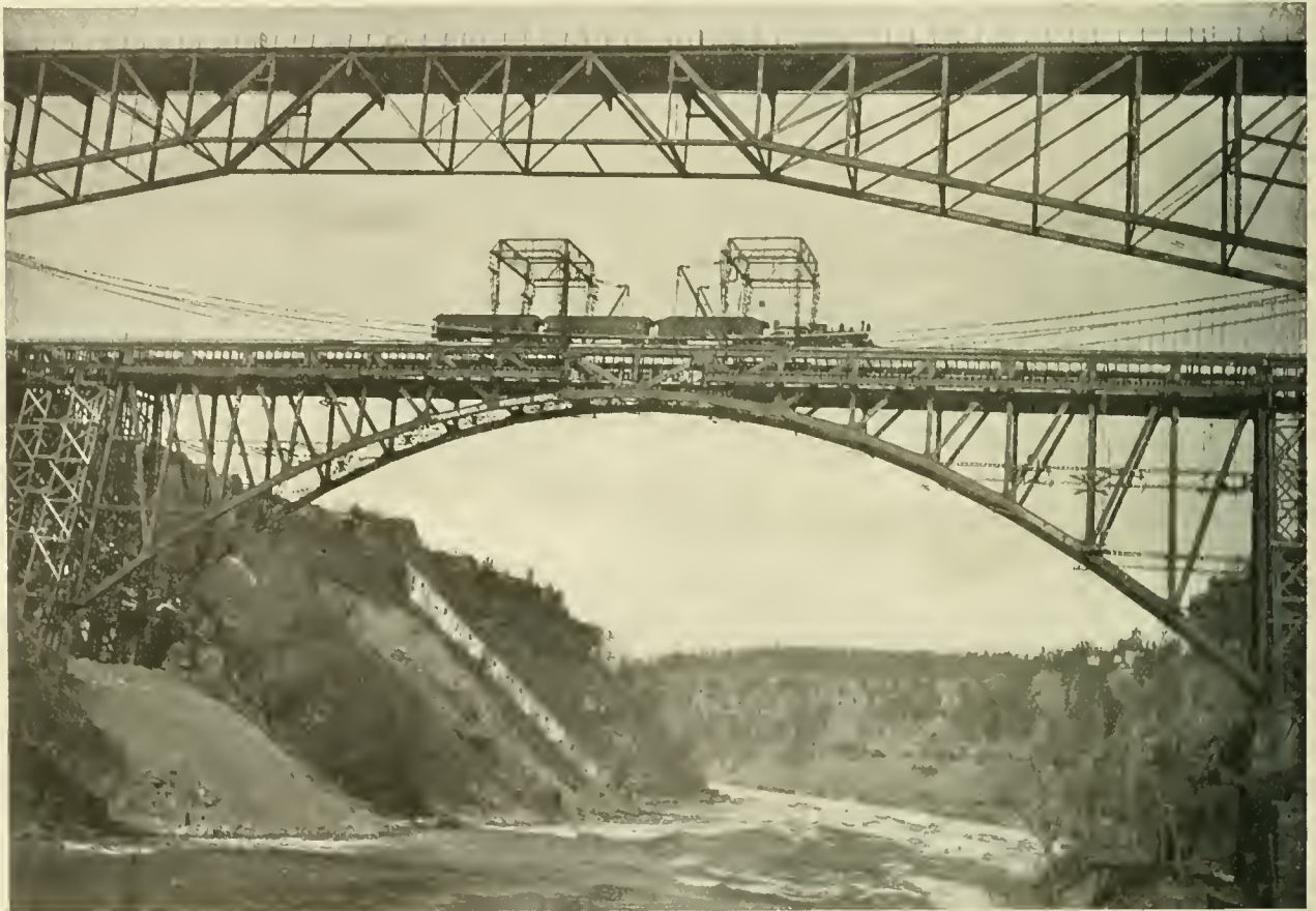
NEW BRIDGE OVER NIAGARA RIVER.
