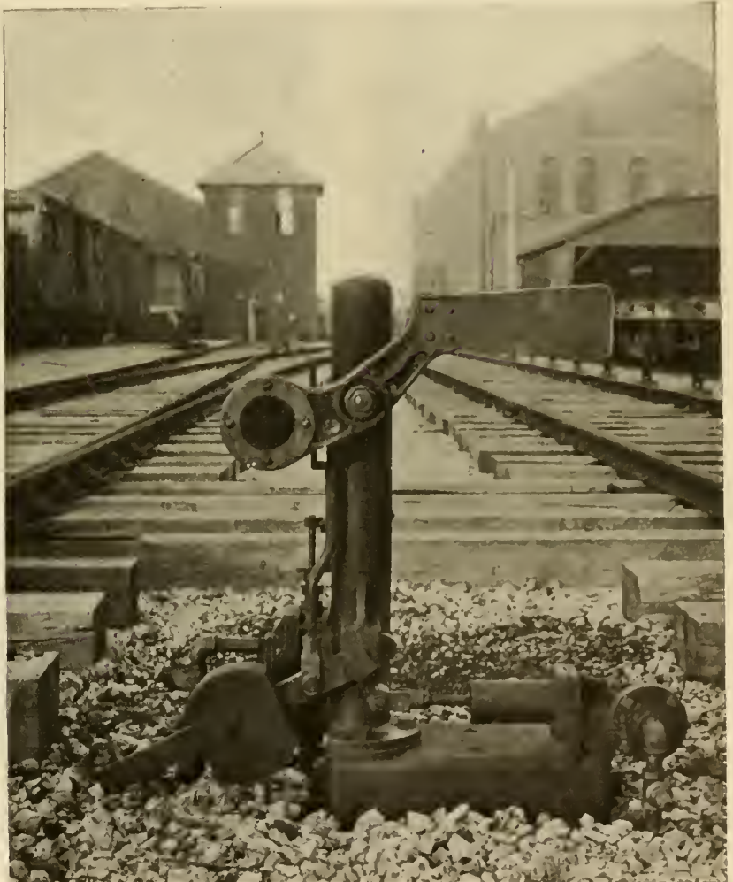
DWARF SIGNAL, CAN BE OPERATED SIXTY TIMES PER MINUTE.
