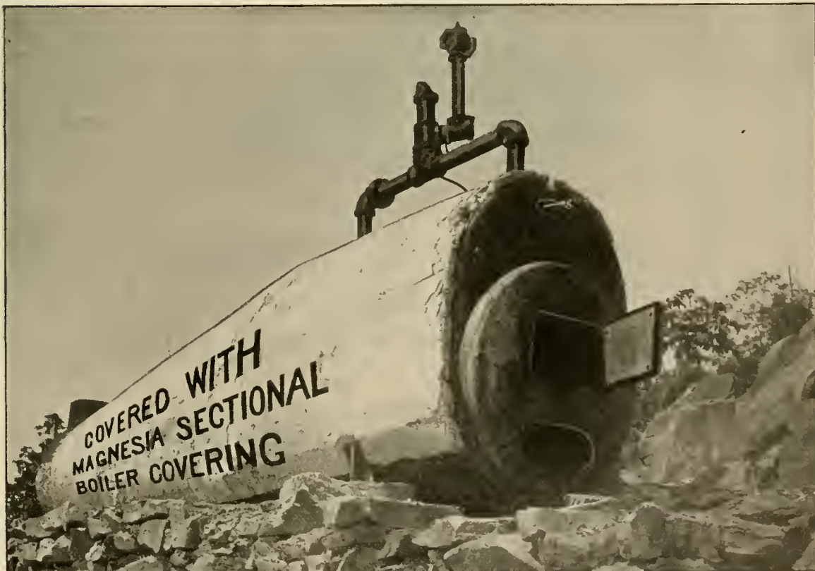
View of boiler of Glen Echo Café, on Conduit Road, Washington, D. C., which was completely destroyed by fire, November 19, 1890. The boiler and steam pipes covered with MAGNESIA SECTIONAL COVERING were the only things saved from destruction. The boiler with the Magnesia still intact, has been continuously and completely exposed to the elements since the fire, now about four years. Both boiler and covering are still in a good condition, and the owners, Messrs. E. & E. Baltzley, propose now to use the old coverings, which have passed fire, water, frost and snow, upon the boilers of the new restaurant. SHOWING FIRE-PROOF CHARACTER OF THE MAGNESIA SECTIONAL COVERINGS.
