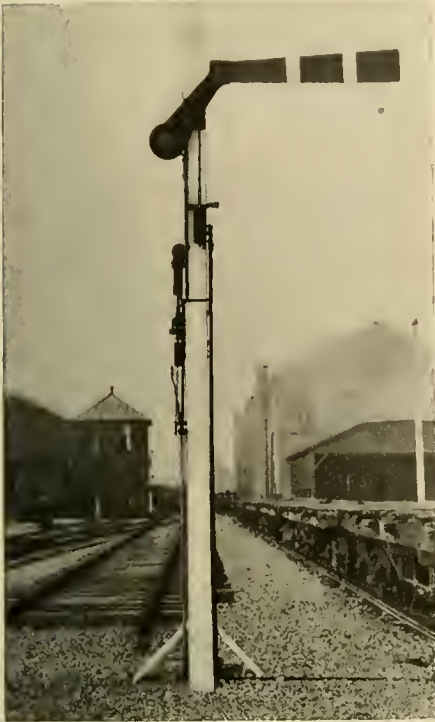
TWO-POSITION SIGNAL, SHOWING SIGNAL INDICATION VALVE.
