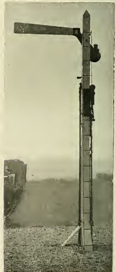
REAR VIEW OF TWO-POSITION SIGNAL.
