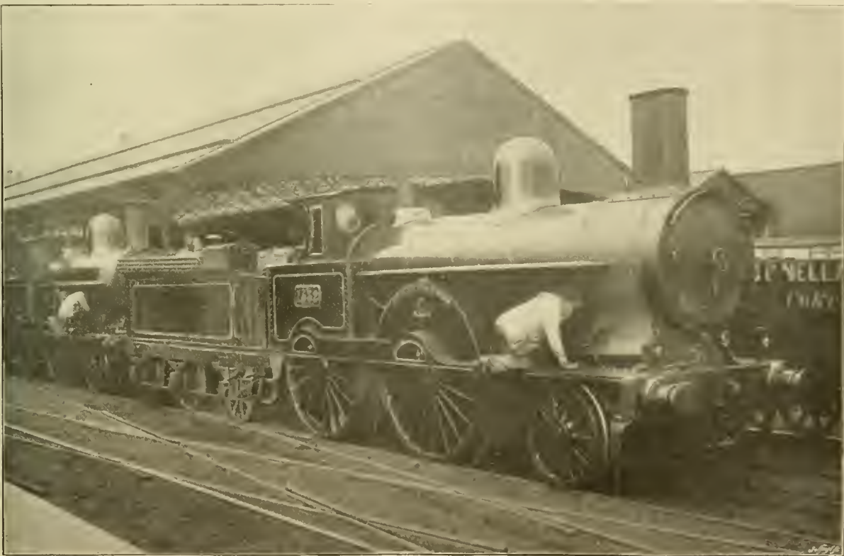
ENGINE WITH DOUBLE STACK—LONDON & NORTHWESTERN RAILWAY.
