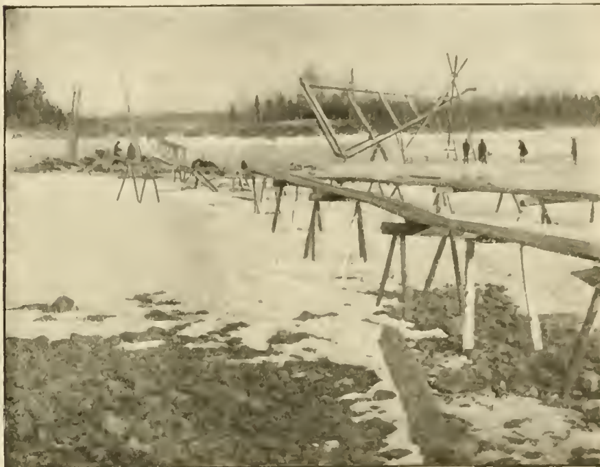
BRIDGE BUILDING. TAKING SOUNDINGS THROUGH THE ICE.
