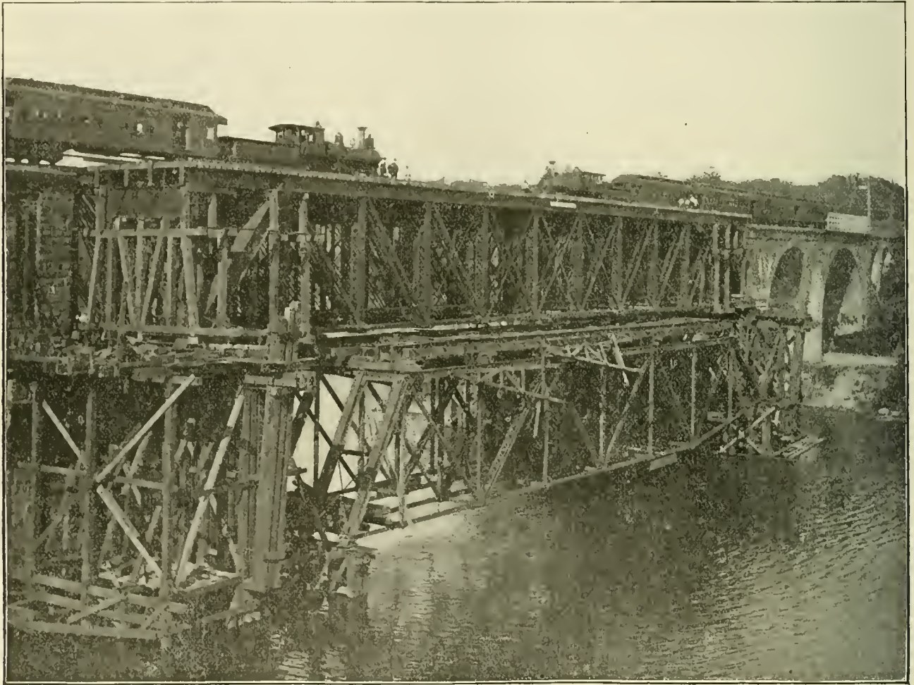
BRIDGE READY TO MOVE INTO PLACE.
