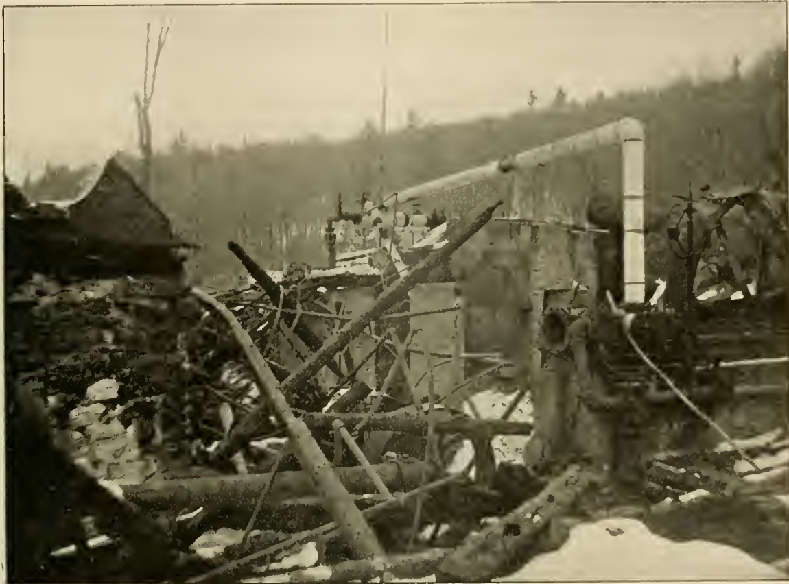
Ruins of the A. W. Eaton Paper Co.'s Mill, at Lee, Mass. SHOWING FIRE-PROOF CHARACTER OF THE MAGNESIA SECTIONAL COVERINGS.
