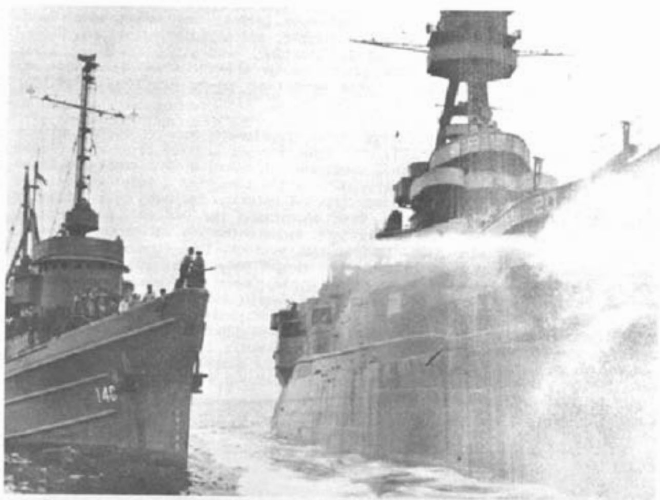
Figure 34. USS Achomawi (ATF-148) spraying USS New York (BB-34) with saltwater after BAKER, CROSSROADS.
