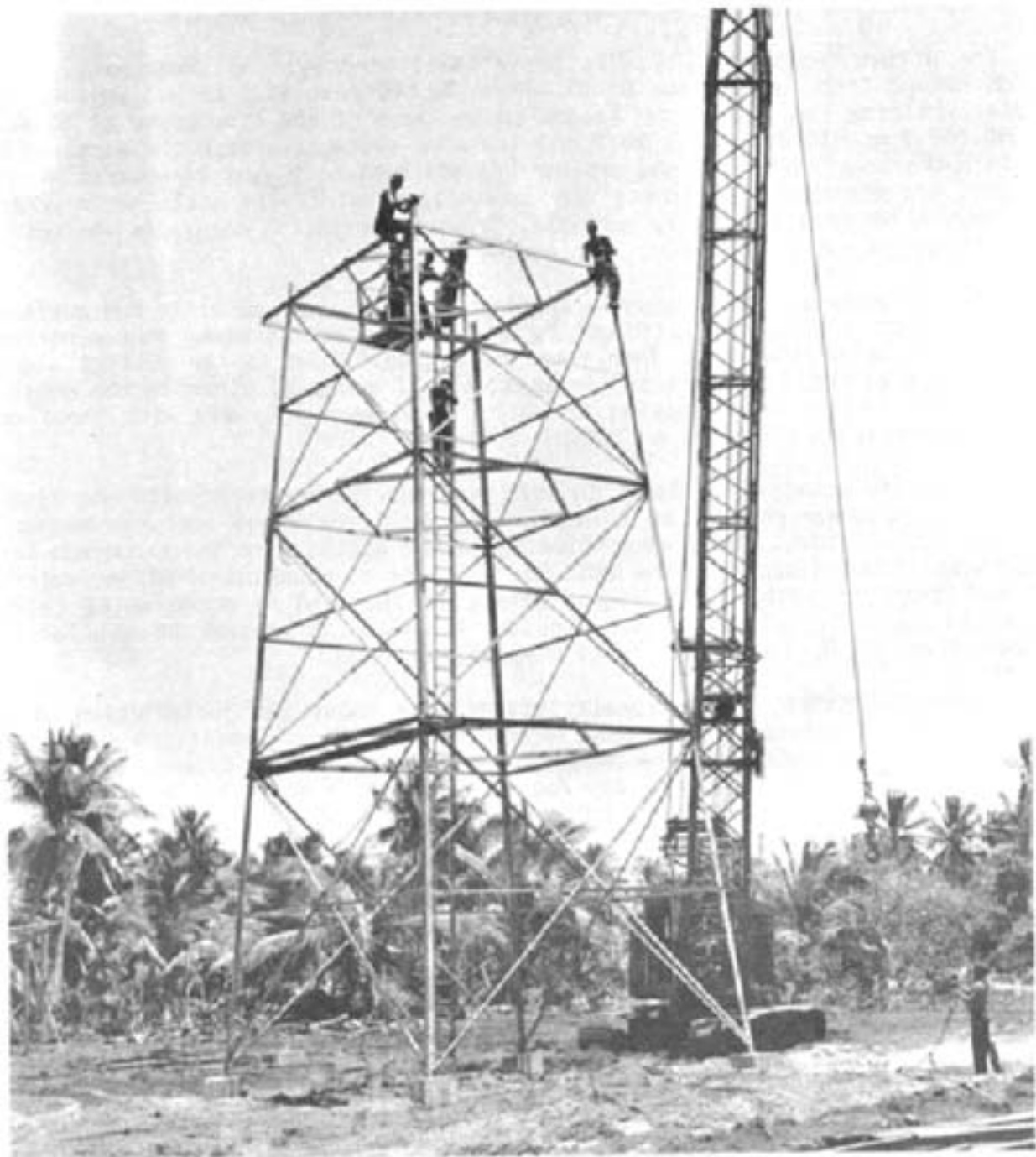
Figure 7. Erection of photo towers on Bikini, prior to CROSSROADS, 1946.
