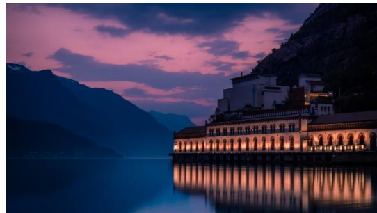
10th place: Early morning at Tyssedal hydroelectric power plant. Photo: Jorulf Kyrkjeide. CC BY-SA 4.0.
