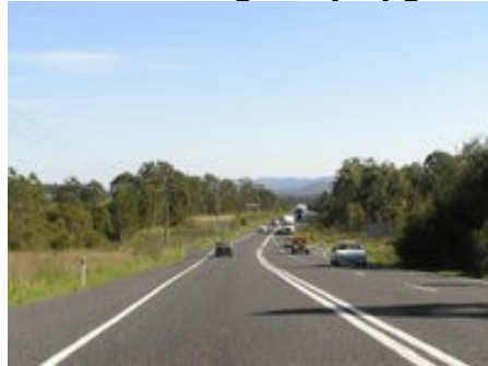
A section of the Pacific Highway South of Buladelah
