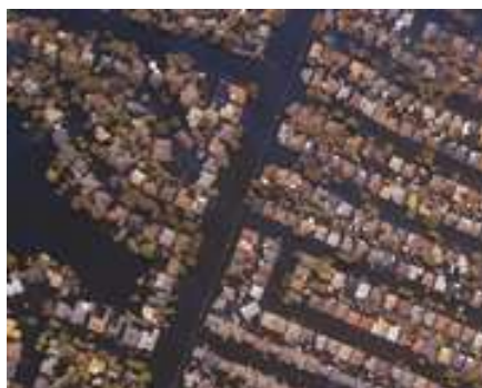
Flooding of residential areas
