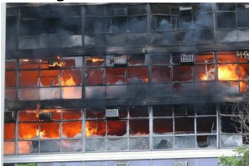
Brasília, Brazil - An building of the Social Security Ministry (INSS) in
