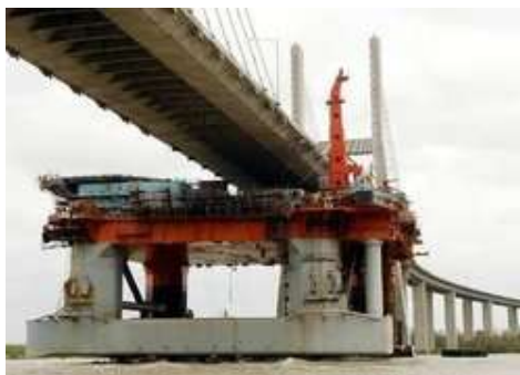
Oil rig platform hits a bridge in Mobile Bay
