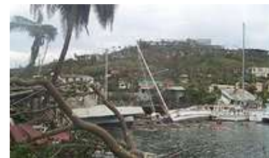
The damage after Hurricane Ivan in 2004
