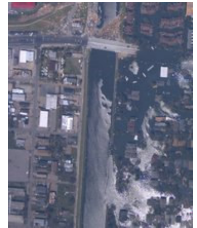
Breach in 17th Street Canal flood wall in New Orleans, Louisiana, August 31, 2005. (NOAA)
