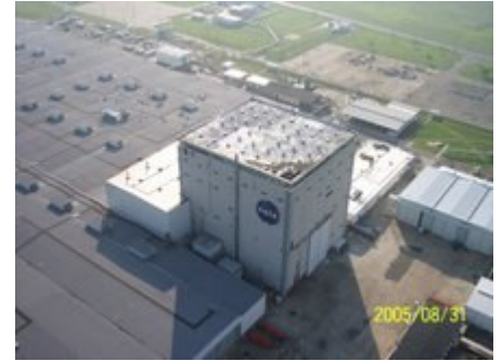
Damage at Michoud Assembly Facility
