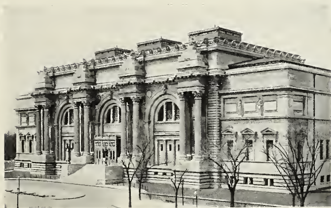
EAST WING OF THE MUSEUM AS COMPLETED
