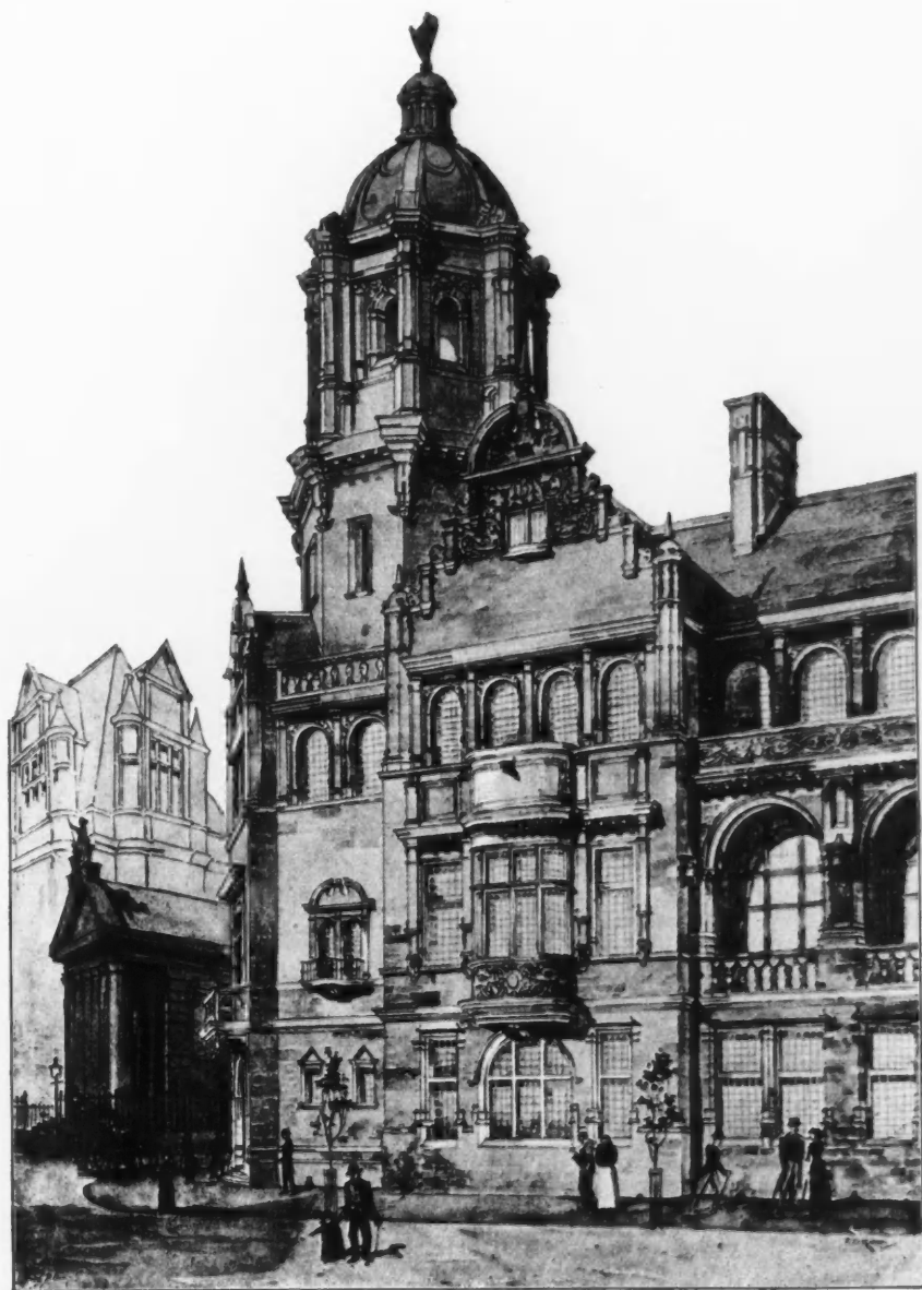
1628. Bond Street Façade, County Council Offices, Wakefield, GIBSON AND RUSSELL, Architects.
