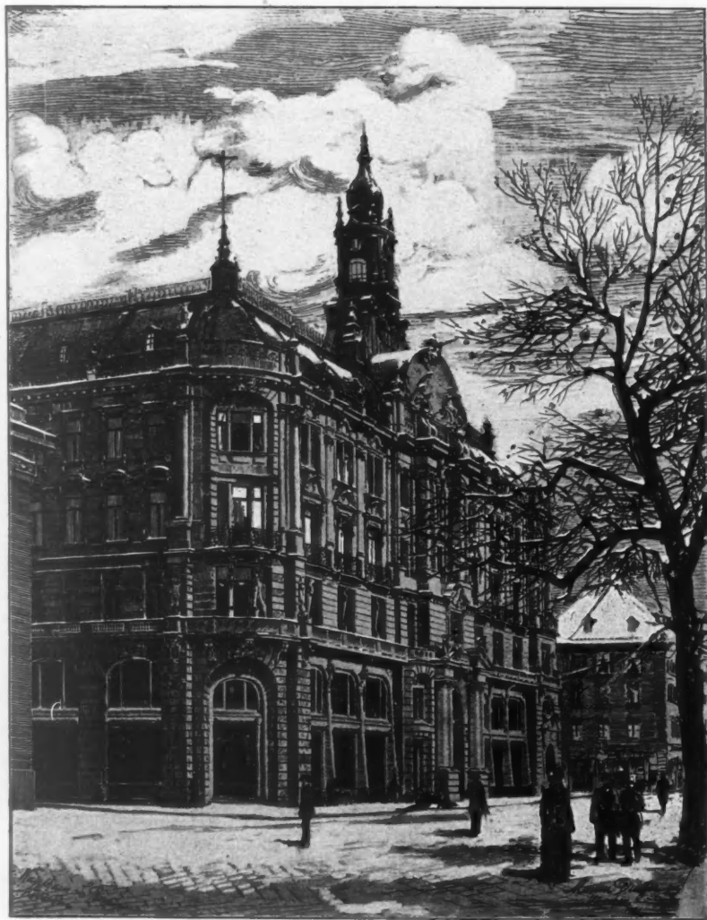
Business Premises and Dwelling House of L. Bernheimer, Commerzienrath. Maximiliansplatz, Munich, PROFESSOR FRIEDRICH THIERSCH AND MARTIN DÜLFER, Architects, Munich.
