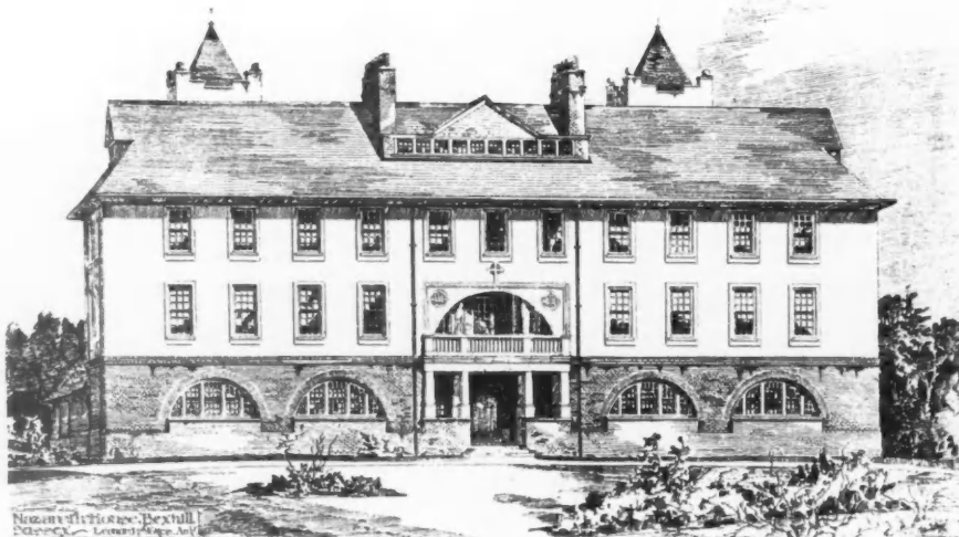
1597. Nazareth House, Bexhill , LEONARD STOKES, Architect.
