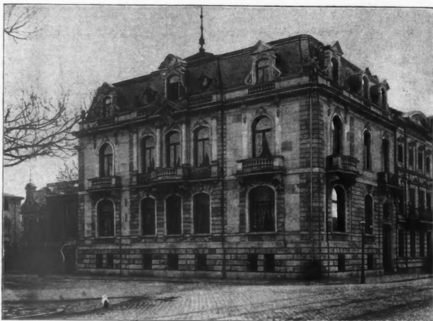
House at Düsseldorf for Herrn Franz Haniel, KAYSER AND VON GROSZHEIM, Architects, Berlin.
