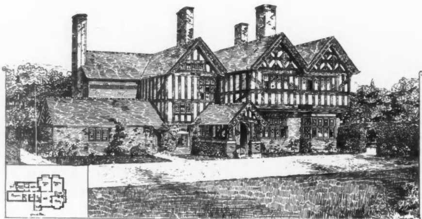
1604. House recently built at Douglas, MACKAY H. B. SCOTT, Architect.
