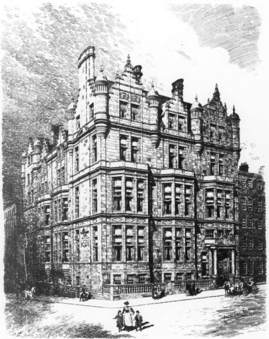
1539. New Club House, for Conservative Club, Glasgow , ROBERT W. EDIS, F.S.A., Architect.
