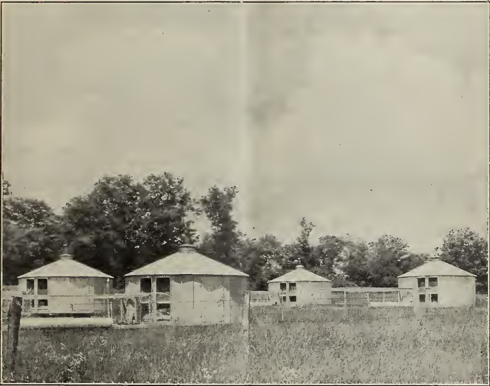
The people who live in modern fabricated steel houses have nothing on the turkey poulters these days! Pictured above are the new steel brooder houses which have received such popular acceptance among progressive growers. Made of fireproof steel, well insulated, and thoroughly engineered for proper ventilation and avoidance against drafts, these new poult houses are sanitary, warm and dry, and effective proof against rats and weasels. (Photo courtesy Martin Steel Products Co.)
