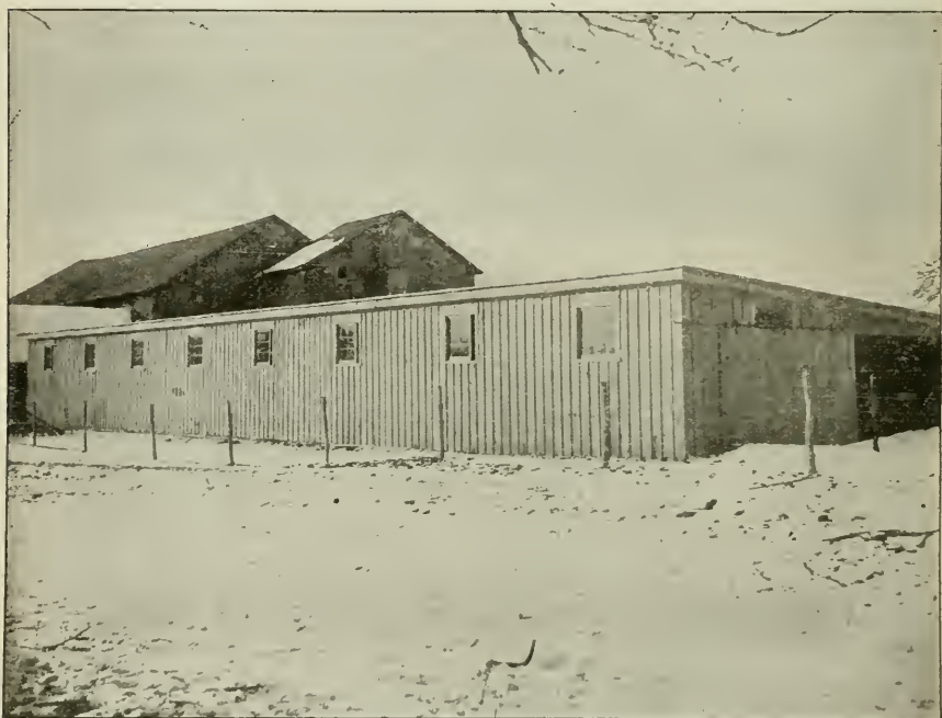
FIG. 332.—Covered barnyard recently built by Clayton Taylor, Lawton Station, N. Y. Twelve-foot post on one side and eight-foot post on the other side.
