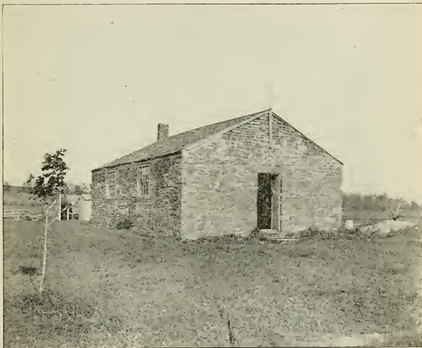
FIG. 139. Substantial but bare. The picturesque finish of vines is needed.
