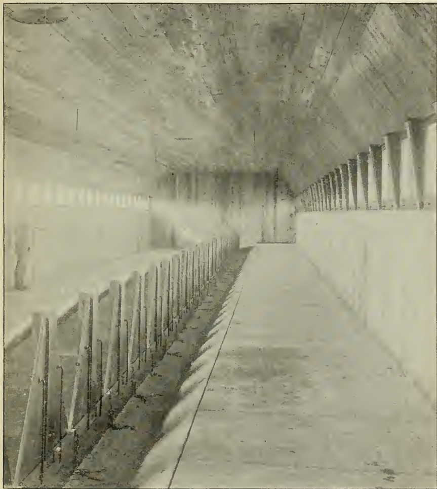
FIG. 327.—A convenient and sanitary arrangement for cow stables. Position of floor in feed alley not inconvenient and saves one foot in height of outside walls. All woodwork has been planed and treated with two coats of boiled linseed oil. See also Fig. 326.
