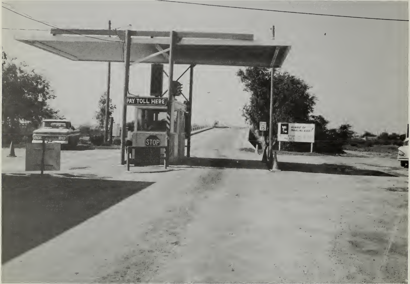
Port of Entry and International Bridge at Nuevo Progreso.
