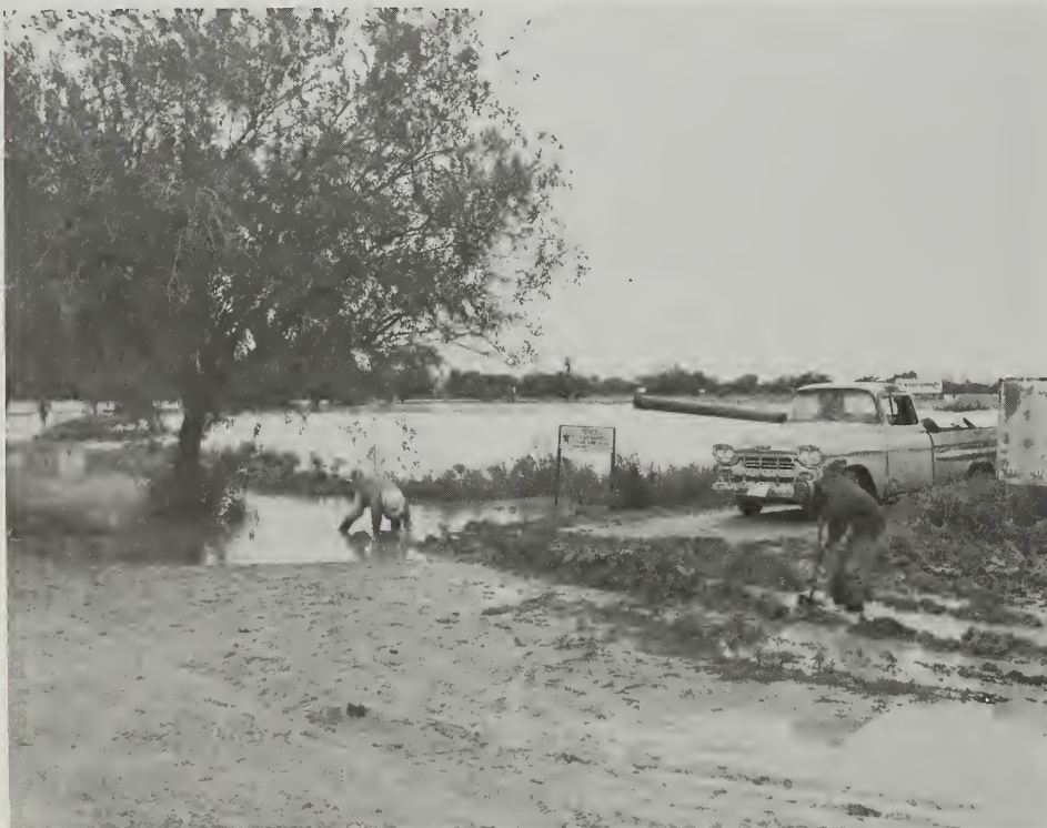
Inadequate drainage structures under roads and railroads cause prolonged flooding. (May 1963)
