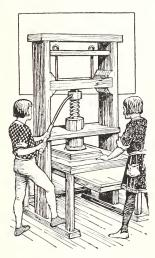
Germany, in 1456. Gutenberg's first types were small blocks of wood. Shortly after, he used the wood type as a pattern for a plaster mold, and then cast pieces of type by the hundreds from such molds. The metal type could be set together to print any page and then taken apart and used again.
