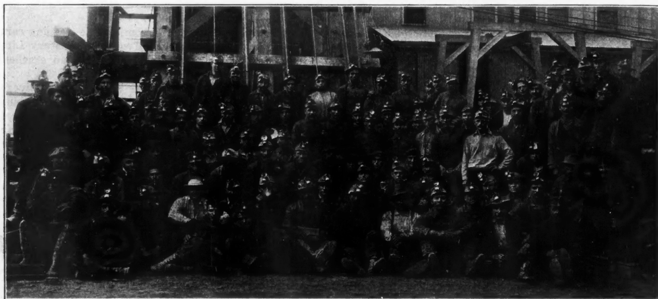
PART OF CREW AT REPLOGLE MINE AT COLLAR OF MAIN SHAFT. RECONSTRUCTION OF HEADFRAME TO PERMIT HOISTING FROM THREE COMPARTMENTS UNDER WAY (NOW COMPLETED)
