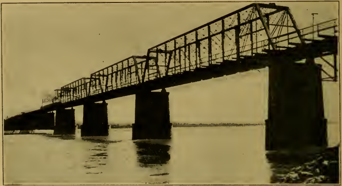
FIG. 72. UNION PACIFIC BRIDGE AT OMAHA
