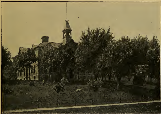
FIG. 76. A TYPICAL TOWN SCHOOL GROUND AND BUILDING, FLORENCE, NEBRASKA
