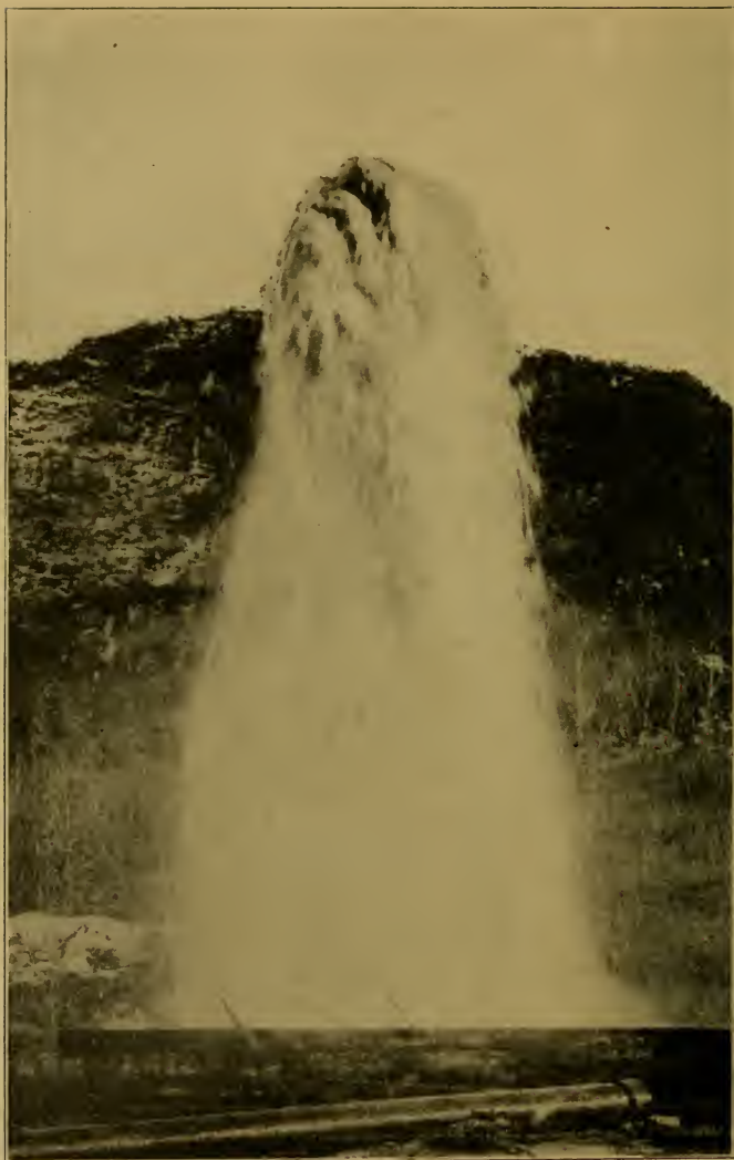
FIG. 15. THE DEEP ARTESIAN WELL AT LYNCH, NEBRASKA THROWING WATER 20 FEET IN THE AIR BEFORE IT WAS USED FOR MILL POWER.
