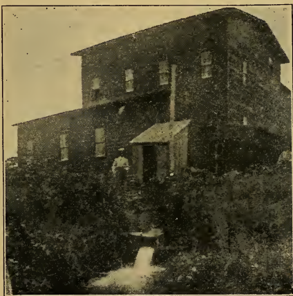
FIG. 16. THE NIOBRARA FLOURING MILL OPERATED BY WATER FROM AN ARTESIAN WELL, THE OVERFLOW OF WHICH SHOWS IN THE FOREGROUND
