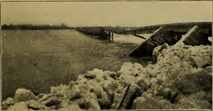
FIG. 24. RAILROAD BRIDGE AT SOUTH BEND DAMAGED BY ICE GORGE
