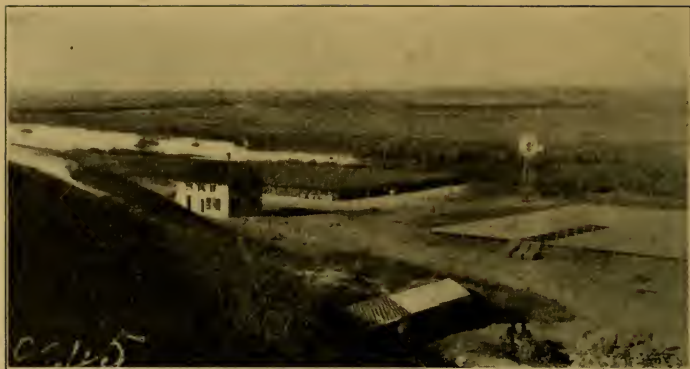
FIG. 112. GENERAL VIEW OF SEED BEDS AND BUILDINGS AT THE DISMAL RIVER FOREST RESERVE, NEAR HALSEY
