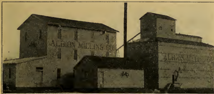
FIG. 99. FLOURING MILL AT ALBION
