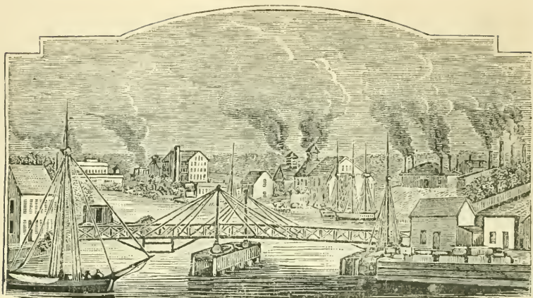
Southern View of Millville, N. J., near the Bridge.
