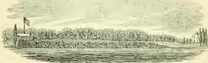
Red Bank, from the Delaware River.
