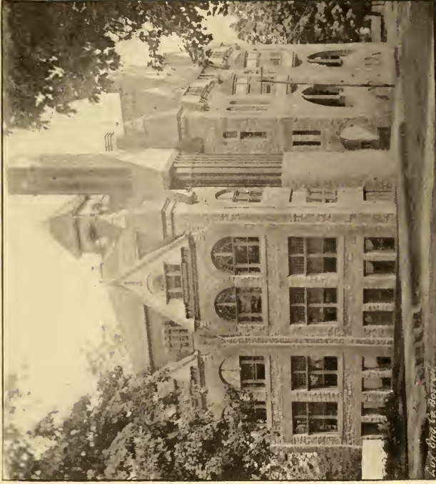
DOYLESTOWN PUBLIC SCHOOL BUILDING.
