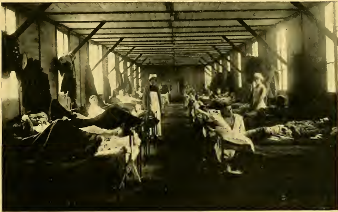
INTERIOR OF ADRAIN BARRACKS USED FOR OVERFLOW OF PATIENTS.
