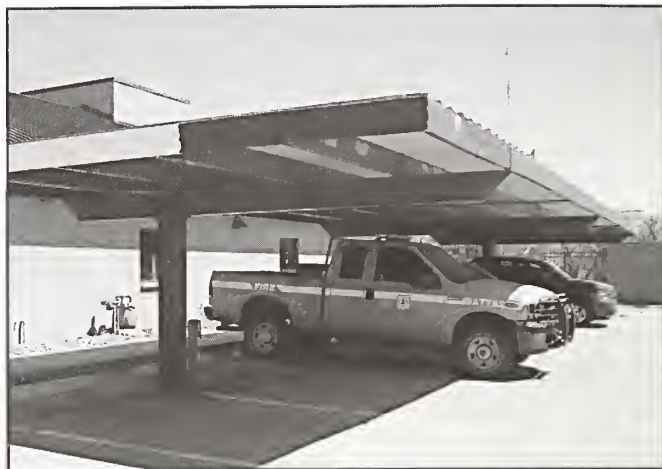
Figure 4—Vehicle exhaust could be drawn into a building's HVAC system if a carport is near the air intake. The air intake for this building is on the roof to prevent vehicle exhaust from being drawn into the Nogales Ranger Station of the Coronado National Forest in the Southwestern Region.
