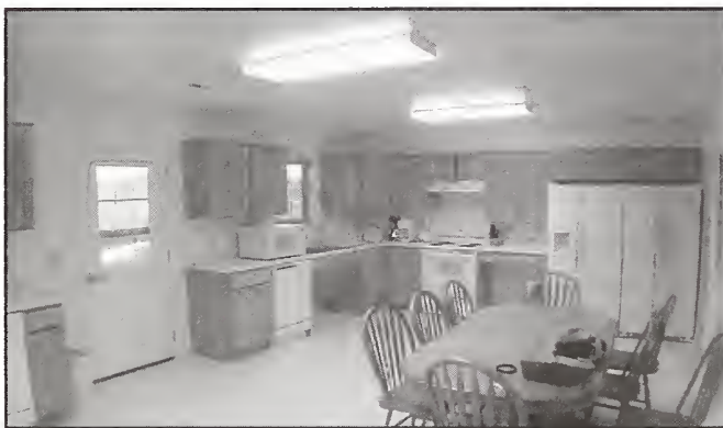
Figure 2—New cabinets, such as those in this bunkhouse, are sometimes the source of chemicals that offgas, contributing to poor indoor air quality and possibly causing headaches or throat and eye irritation.
