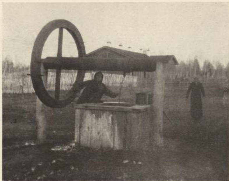
WELL AT KHUVOELANSKAYA STATION (OCT. 20)
