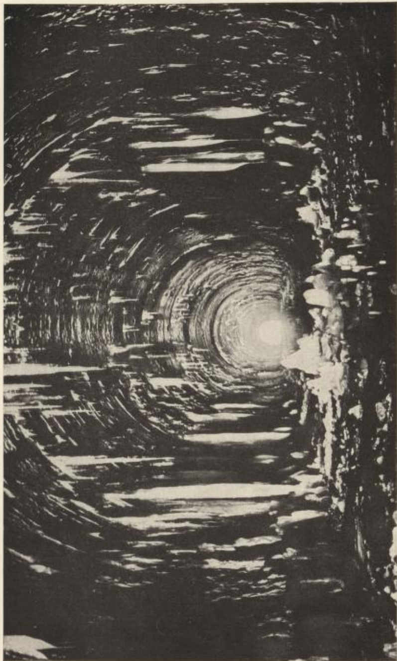
A FOEN TUNNEL ON THE AMUR RAILWAY
