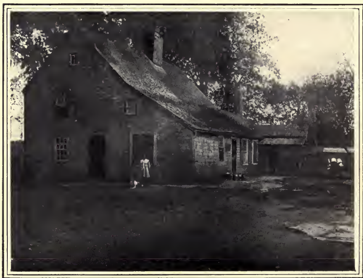
The Kingsley Lean-to, South Rehoboth. Residence of Harlan P. Wyman, Esq.
