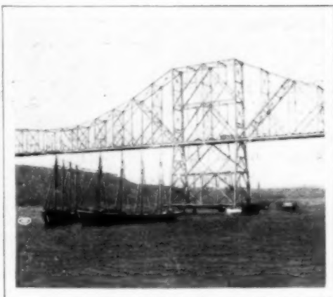
Old Wooden Ships Guarding the Central Pier of Big Steel Bridge from Damage by Collisions
