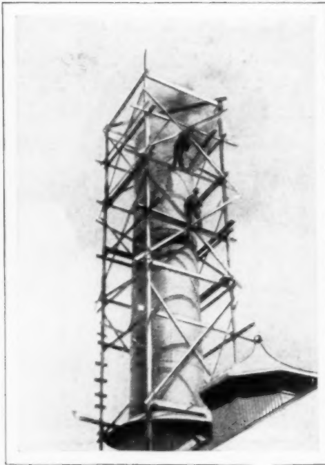
Adding Section to Big Smokestack While Fires Burned Below; Workmen Completing Second Half of a Joint
