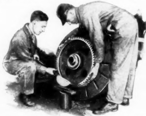
Pouring Lead around Rim of Street-Car Gear Wheel, to Help Deaden the Noise
