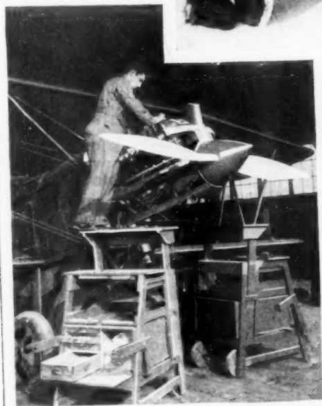
Each Pursuit Ship Has Its Own Crew of Mechanics to Keep It Flying; Center, Changing from Wheels to Skis for Winter Work
