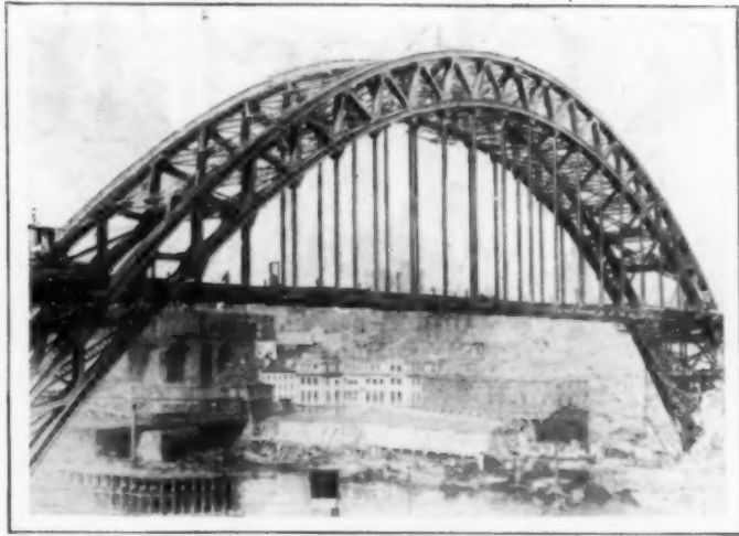
Long Span of the Tyne Bridge between Newcastle and Gateshead, England; the Structure Cost Nearly $5,000,000
