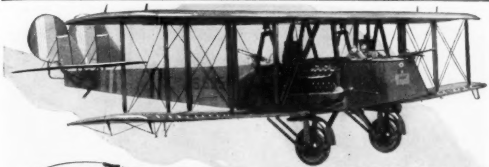
The Army's Latest Twin-Engine Curtiss Bomber; Instead of a Third Engine in the Nose It Carries a Machine Gunner There, While Another, behind the Pilot, Fires toward the Rear, and the Bomber Drops His Missiles through the Floor; Left, a 4,000-Pound Bomb
