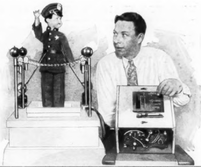
Model of Dummy Policeman and Traffic Lights for Installation at Intersections, to Replace a Human Attendant
