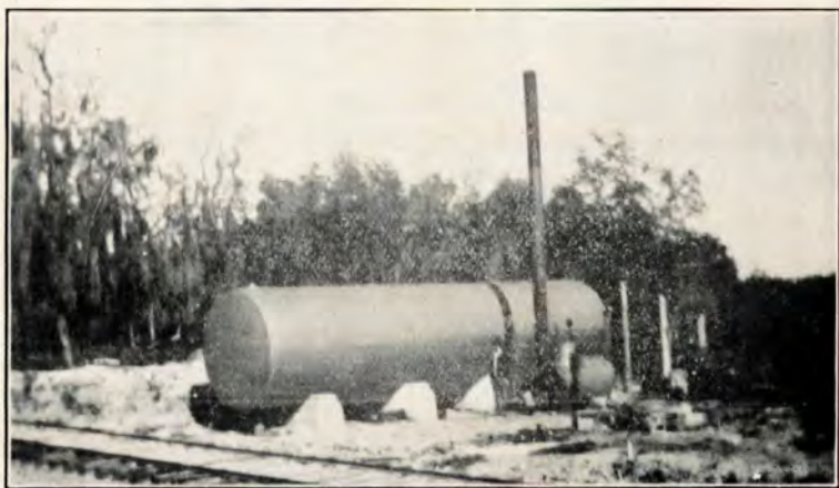
THE NEW PUMPING PLANT
