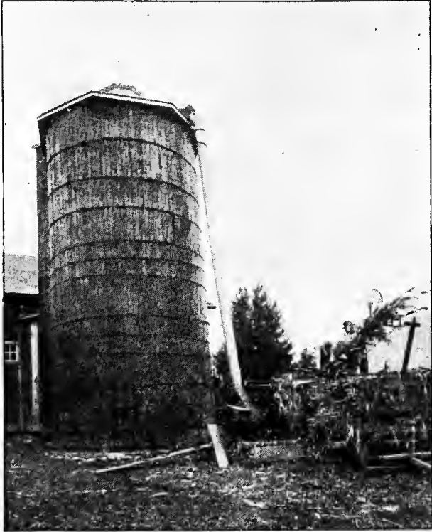
Fig 43—Filling Silo with Blower
